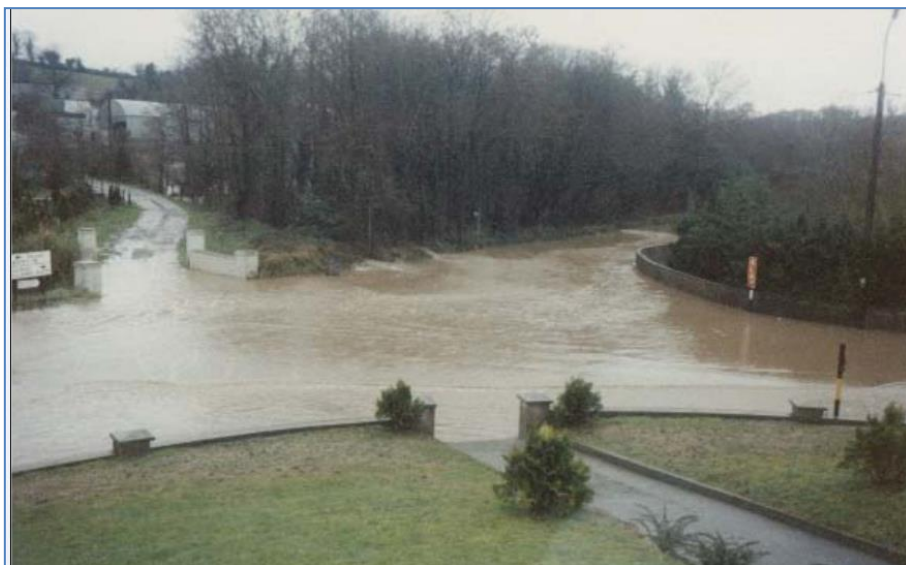
Figure 1.6 - View from St Senan's Church (ref: OPW floodinfo.ie, 6/Feb/1990)
